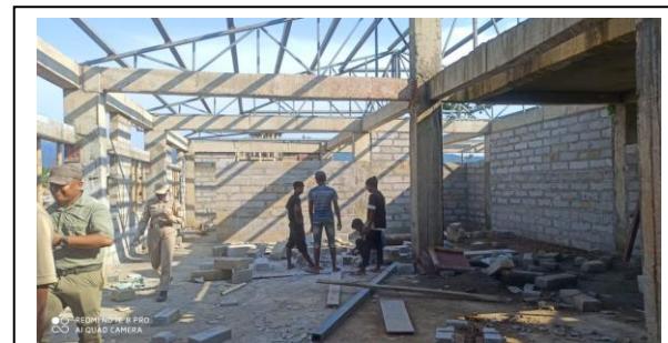
Undergoing construction sites in indoor sports complex
