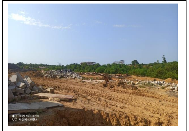
Levelled Parade Ground site
