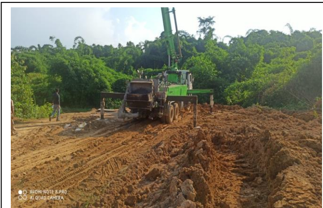
Undergoing construction of the approach road
