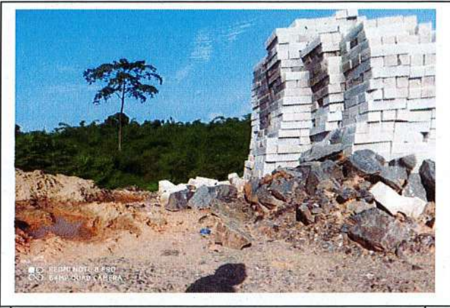
Brick block material inside the proposed site
