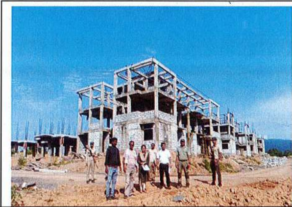
Construction site of Commandant Office Block
