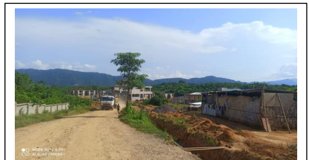
Boundary wall and proposed site
