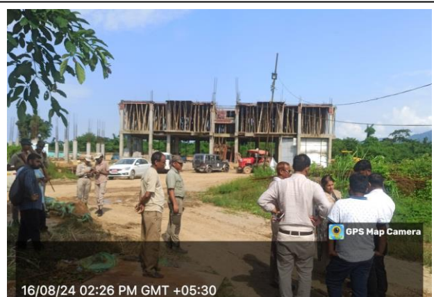
Construction site of Assistant Commandant Block
