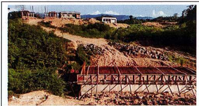
Under construction of culvert for the approach road
