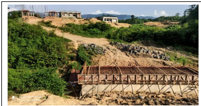
Under construction of culvert for the approach road
