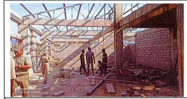
Undergoing construction sites in indoor sports complex
