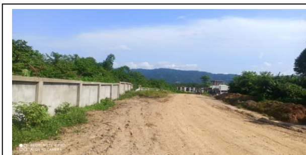
Constructed Boundary wall of the proposed site
