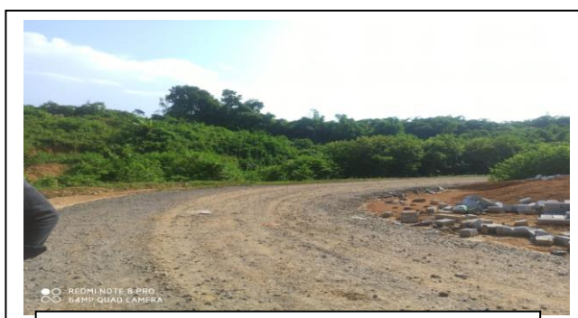
Constructed road inside the proposed area
