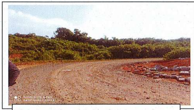
Constructed road inside the proposed area
