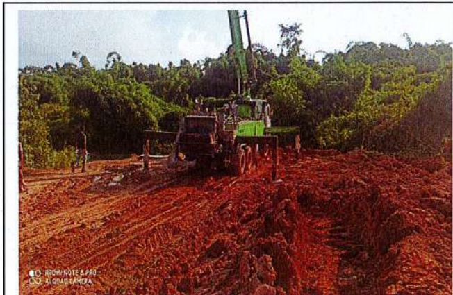
Undergoing construction of the approach road
